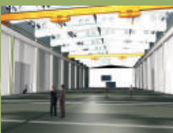
IHI J.V. Factory Made out of IHI Panels & Trusses
