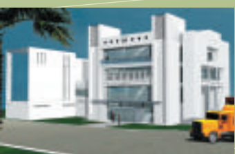
IHI J.V. Factory's Offices
