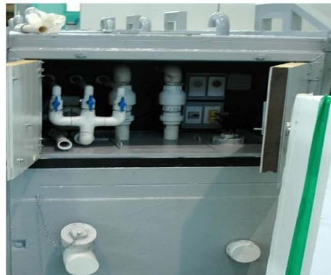
MOBILE INSULATED SEPTIC TANK (PIPING SYSTEM)
