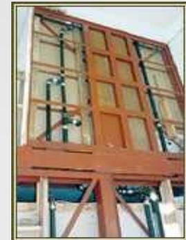
**INTEGRATED WATER/DRAINAGE PIPES INTEGRATED IN THE PANELS
