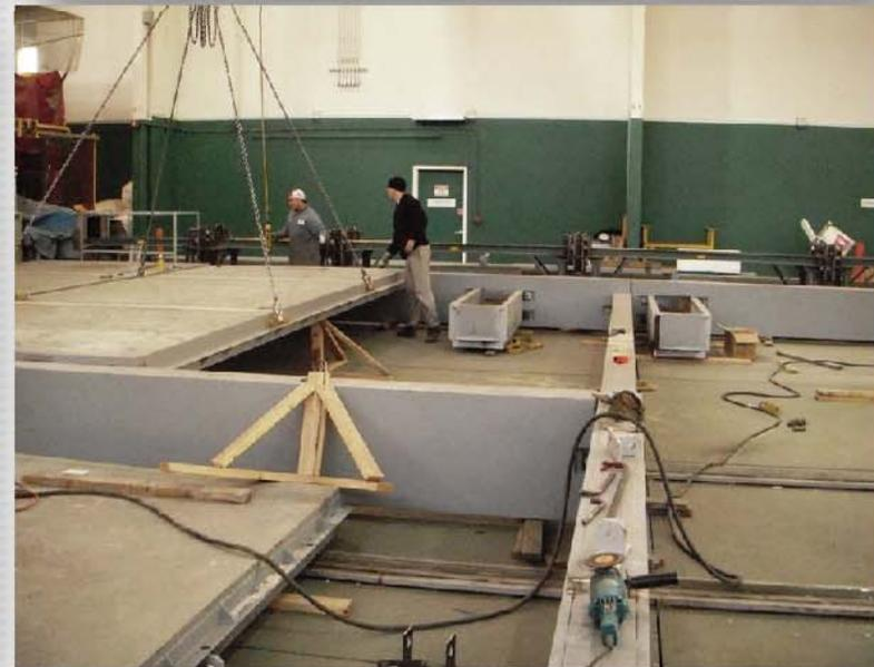
Dry run installation of the IHI foundation and ground floor slab panels. The foundation panels are spanning over few point loads over the IHI facility's raised floor panels. **A further great live test for the superior IHI structural panels that is obviously totally foreign to any other building system in the world including pre-cast and cast in situ systems.**
