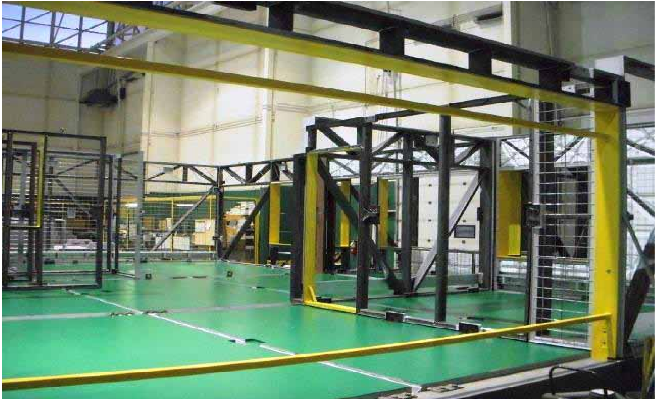
VIEW OF THE TYPICAL UNIT THROUGH THE DINING ROOM VERY LARGE WINDOW SHOWING THE SECOND BEDROOM ON THE RIGHT, THE WINDOW AND DOOR OPENINGS ARE PAINTED IN YELLOW AND THE FLOOR PANELS SEALED IN GREEN.
