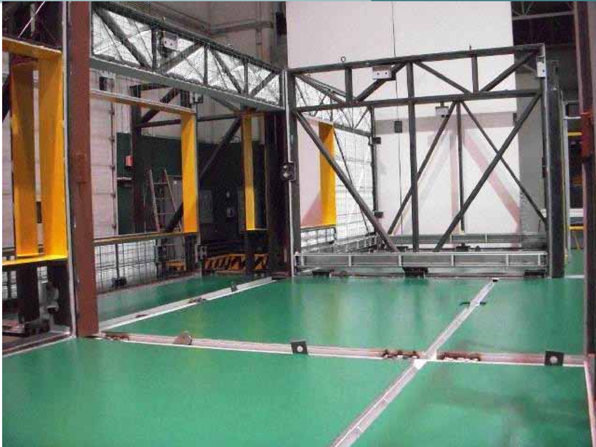
VIEW OF THE LIVING ROOM AREA FROM THE MASTER BEDROOM SHOWING THE WINDOWS (YELLOW) AND THE FLOOR PANELS (SEALED IN GREEN). THE SECOND BEDROOM INTERNAL IHI PANELS AREA SHOWN IN THE BACKGROUND WITH ELECTRICAL CONDUITS/RACEWAYS PLACED AT THE BOTTOM OF THE PANELS.
