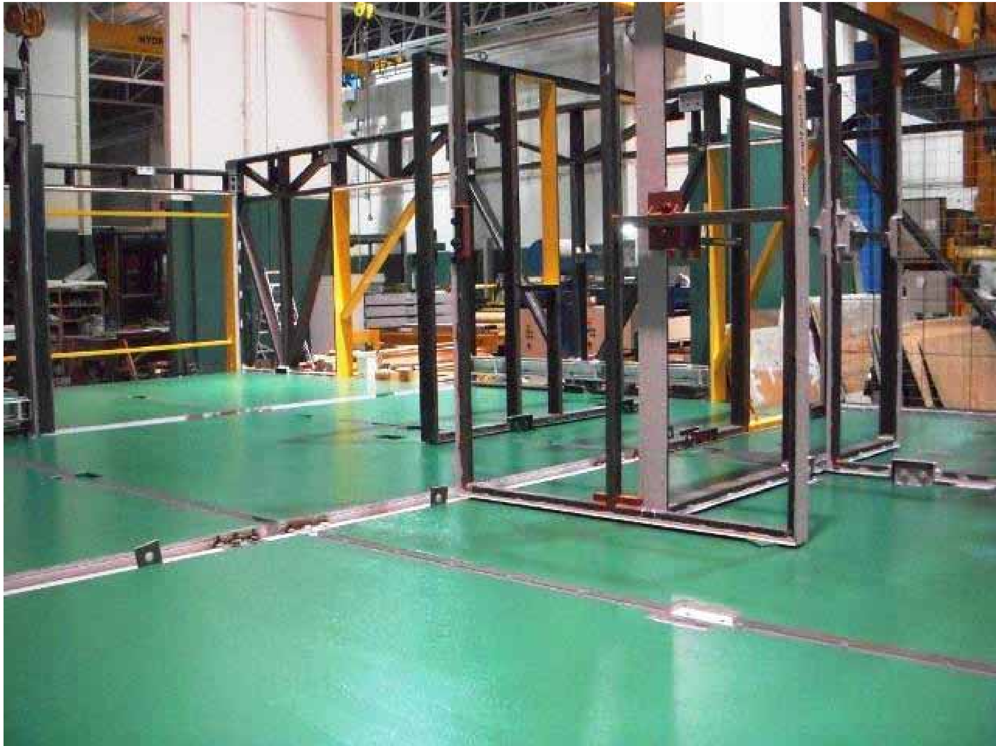
VIEW FROM THE MASTER BEDROOM TOWARD THE RECEPTION AREA WITH THE INTERNAL IHI PANELS IN THE BATHROOM AREA (UPPER RIGHT CORNER). THE PICTURE SHOWS THE PERFECTLY LEVELED SMOOTH FLOOR PANELS ( NO NEED FOR ANY FURTHER LEVELING OR GROUTING) PAINTED SEALED IN GREEN AND READY FOR ANY TYPE OF FLOOR FINISHING.
