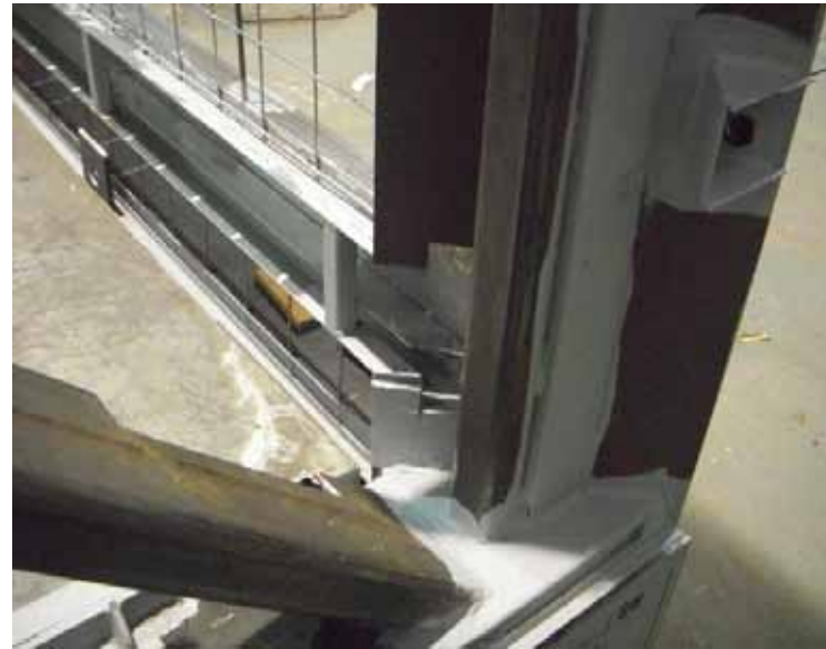
CLOSER VIEW OF CORNER SHOWING DETAIL OF THE TRUSS FOR A PERFECT FIT AND TO OBTAIN SEAMLESS CORNERS AND THE ELECTRICAL CONDUIT CHANNEL RUNNING ALL ALONG THE LOWER END OF THE WALL PANEL.
