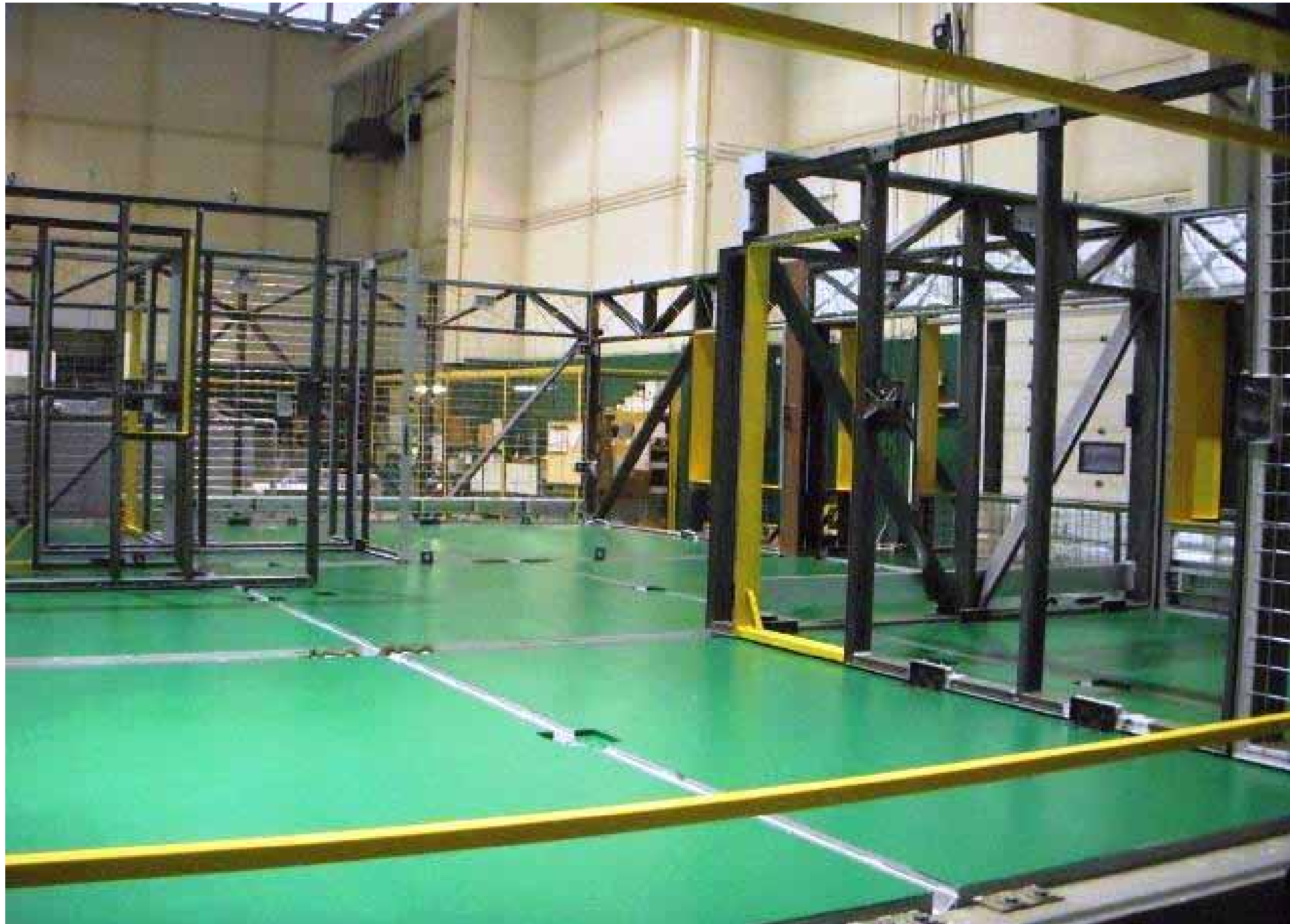
CLOSER VIEW OF THE PREVIOUS SLIDE SHOWING THE KITCHEN/DINING AREA AND SECOND BEDROOM INTERNAL IHI STEEL WALL FRAMES
