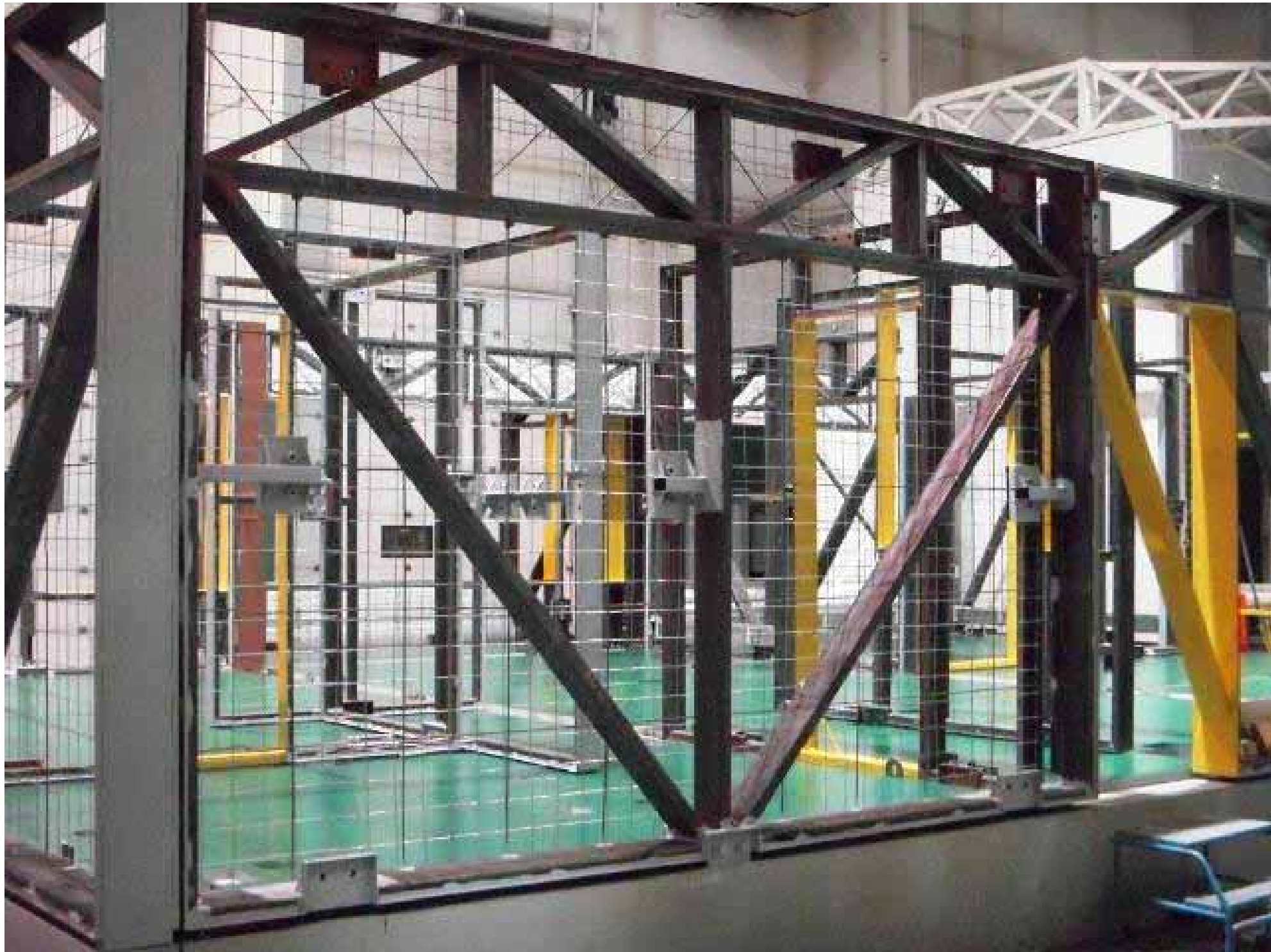
THIS PHOTO SHOWS THE MASTER BATHROOM AREA THROUGH THE EXTERNAL IHI WALL PANELS WITH THE CONTINUOUS STRUCTURAL STEEL TRUSSES THAT WILL BE TOTALLY CONCEALED AFTER CONCRETING THE PANELS. AGAIN, DOOR AND WINDOW HSS SUB-FRAMES ARE SHOWN IN YELLOW.
