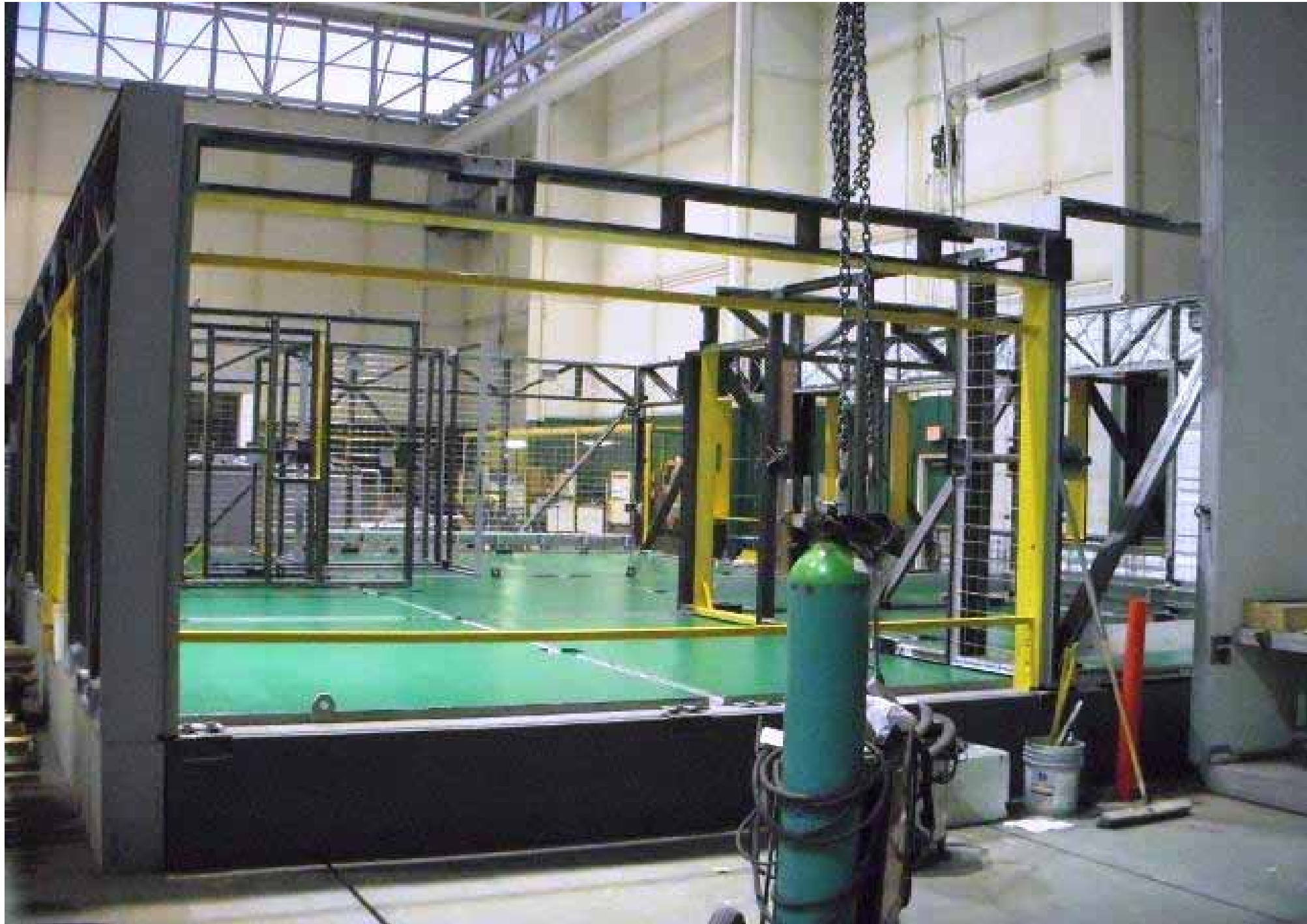
VIEW OF THE FRAME FOR THE VERY LARGE SLIDING DOOR/WINDOW GIVING ACCESS FROM THE DINING ROOM TO THE TERRACE. THE WINDOW HSS CONCEALED SUB FRAME IS PAINTED IN YELLOW AND THE FLOOR PANELS ARE SEALED IN GREEN. THE LONGITUDINAL BRACING WITHIN THE WINDOW SUB-FRAME ARE TEMPORARY (TO MAINTAIN PERFECT ALIGNMENT DURING THE TRANSPORTATION AND ASSEMBLY ) AND WILL BE REMOVED ONCE THE BUILDING IS ERECTED ON SITE.
