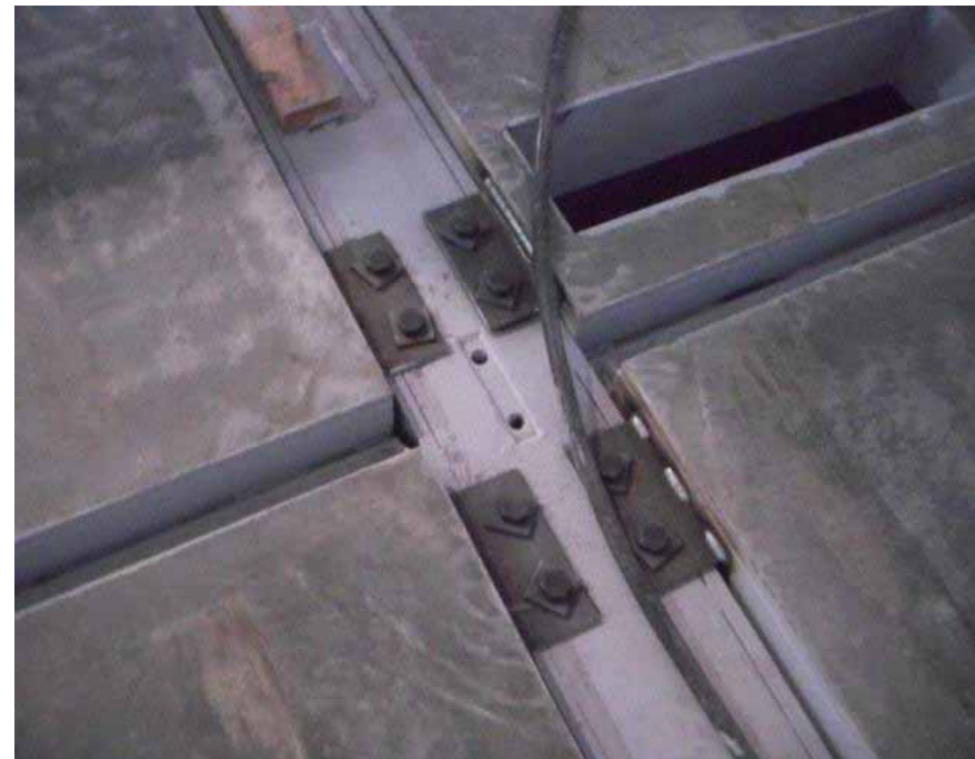
DETAIL OF CONNECTIONS BETWEEN FLOOR PANELS WITH A RECESS TO ALLOW FOR ANY FUTURE MEP UPGRADE
