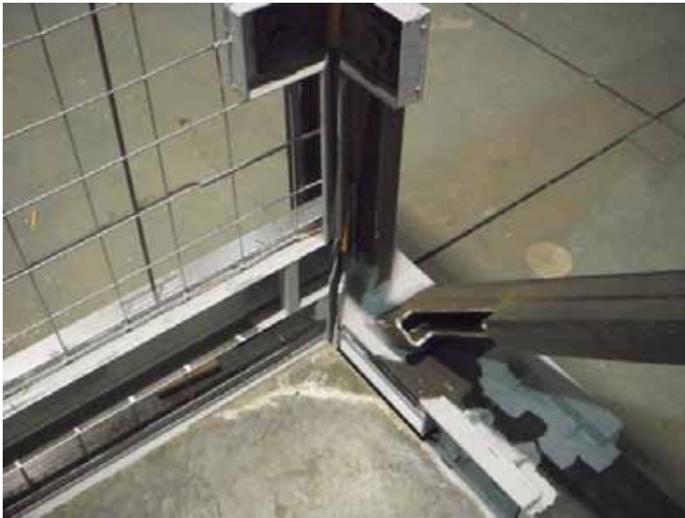
CLOSER VIEW OF CORNER SHOWING DETAIL OF THE TRUSS FOR A PERFECT FIT AND TO OBTAIN SEAMLESS CORNERS AND THE ELECTRICAL CONDUIT CHANNEL RUNNING ALL ALONG THE LOWER END OF THE WALL PANEL.
