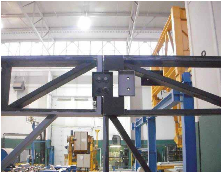
DETAIL OF THE CONTINUOUS TRUSS BEAM CONNECTION
