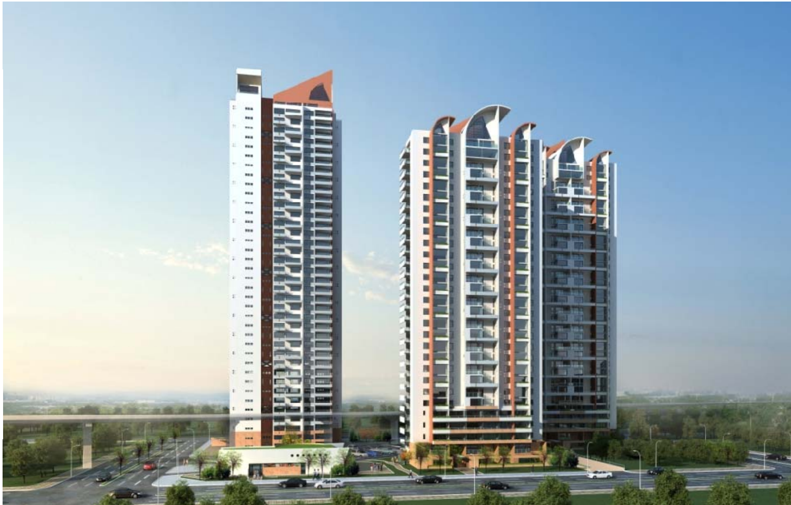
VIEW OF THE PROPOSED OPTIMA 3 TOWERS (AFTER OBTAINING THE HIGH DENSITY THAT IS UNDER STUDY) ALONG UNIVERSITY DRIVE
