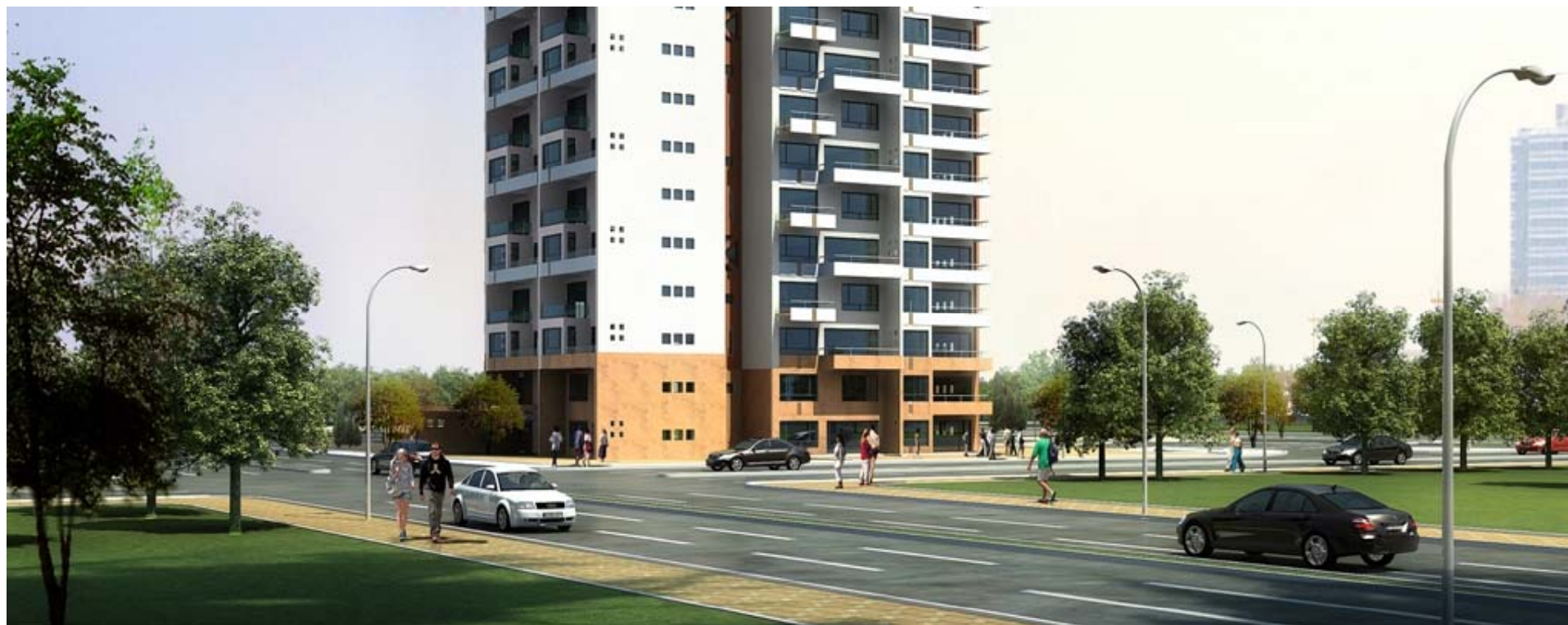
CLOSER VIEW OF MAIN ENTRANCE AND LOWER FLOORS
